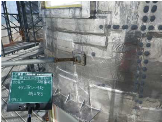
Covered with titanium foils
