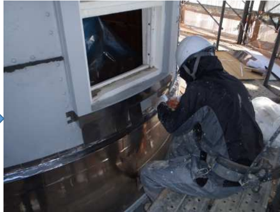
Pre-painting and pasting of titanium foils
